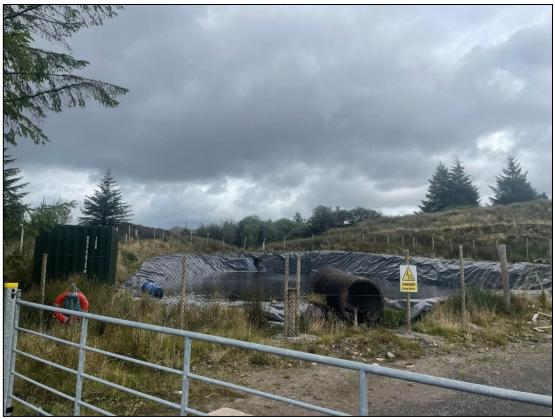
Plate 5-2: Relocated and plastic lined settlement pond showing overflow pipe (August 2023).
