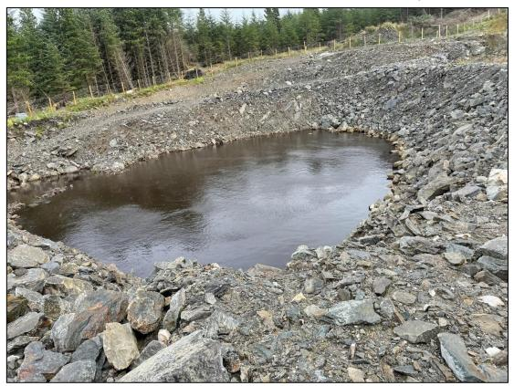
Plate 5-14: Unfilled section of peat cell with artificial pond.
