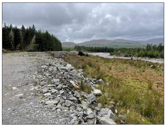
Plate 5-10: Containment berm on left of plate, with amended road to the right. Recolonising habitats visible where conifer forestry has been felled.
