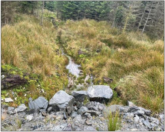
Plate 5-18: Forestry Drain running out of site. Small accumulation of silt at base of bund – no signs of any effects thereafter.
